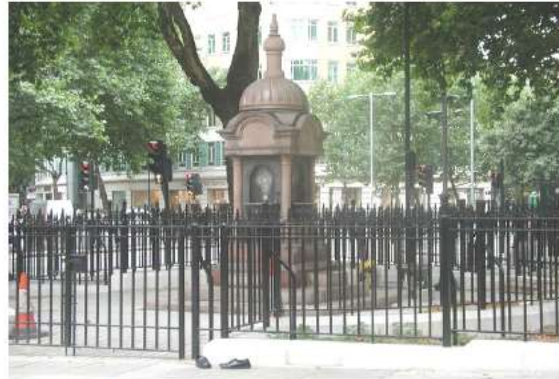
The new fenced and gated site.
